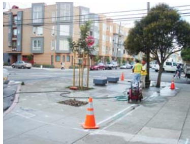
During Concrete Removal
